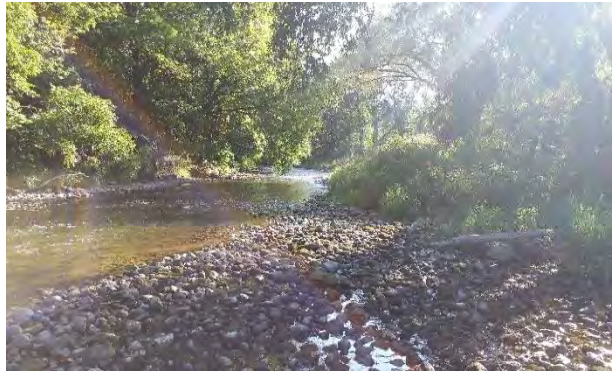
d) S031 outlet at dam looking downstream
