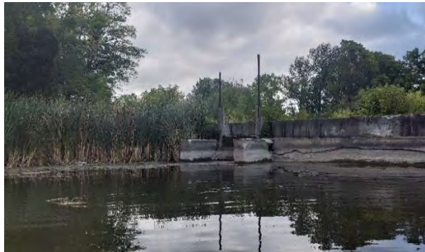
f) Dam at north end of reservoir
