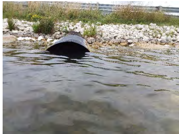
d) Culvert at north end of Hines Lake
