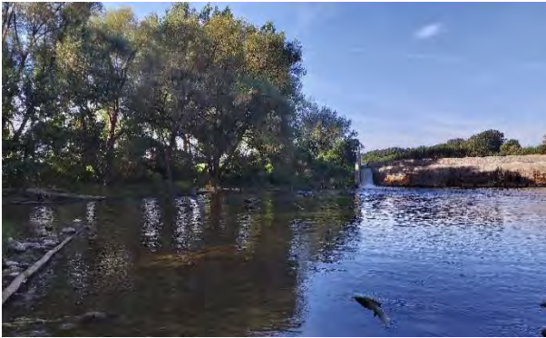
c) Outlet (S031) looking upstream at dam
