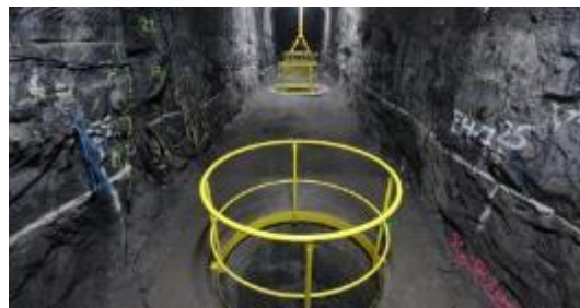
Demonstration facilities –420 m
