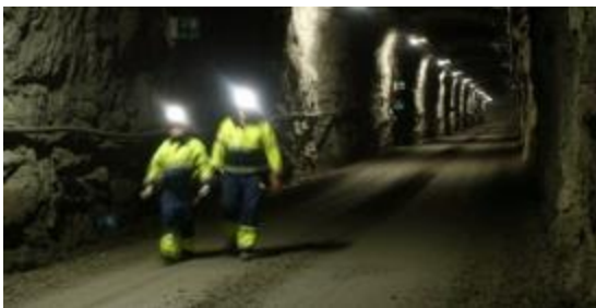
Approx. 6.5 km of excavated access tunnels and vehicle access
