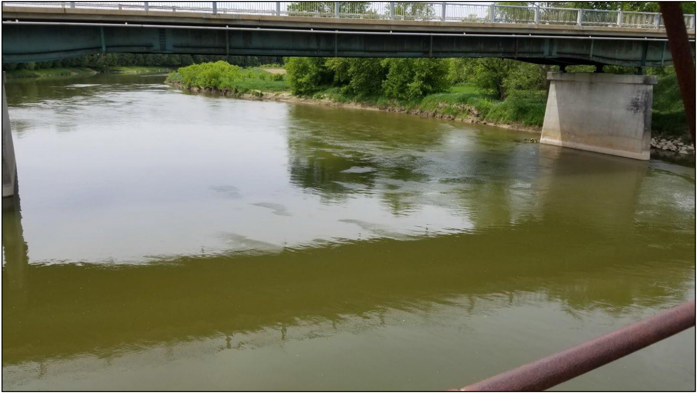
Photo 67. Standing on the pedestrian bridge at SB_SW_Saugeen_01 looking upstream.
