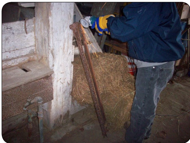
Figure 4. Grinding piece of steel in close proximity to combustible materials.
